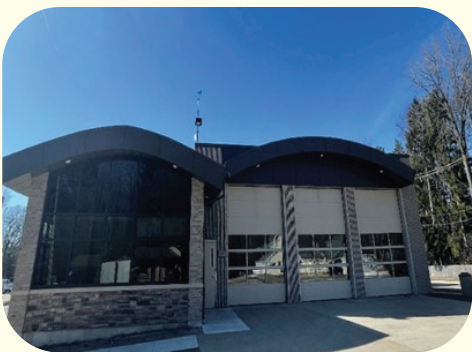
Fire Station #1 Garage
