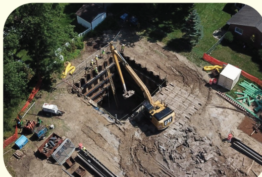
Wet well excavation - Madeline/Sue
