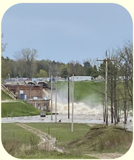
Edenville Dam Break
