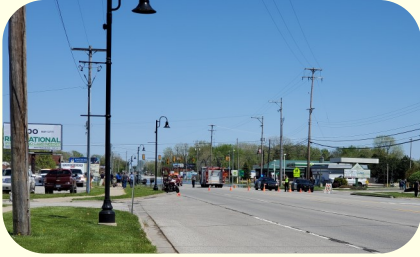
Gratiot Road Bridge closed off due to flooding
