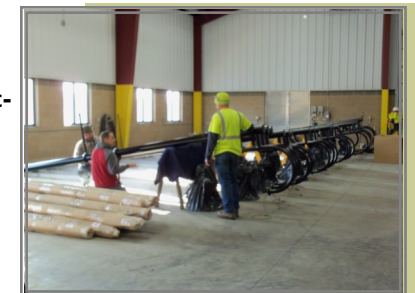
Employees of J. Ranck Electric assemble new lights.
