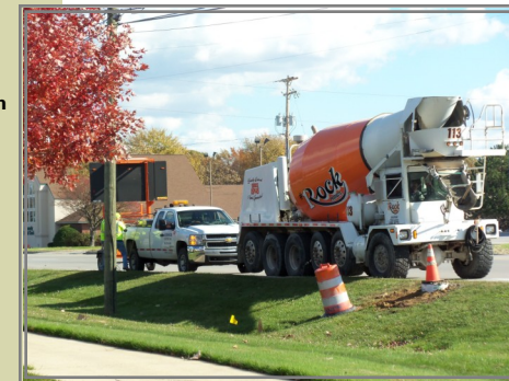
J. Ranck Electric install footings for lights.
