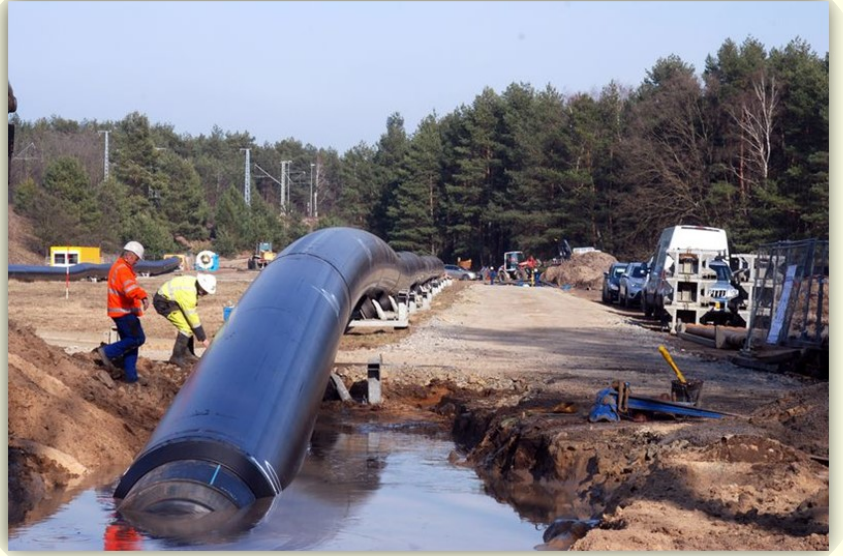
Direction Drilling
