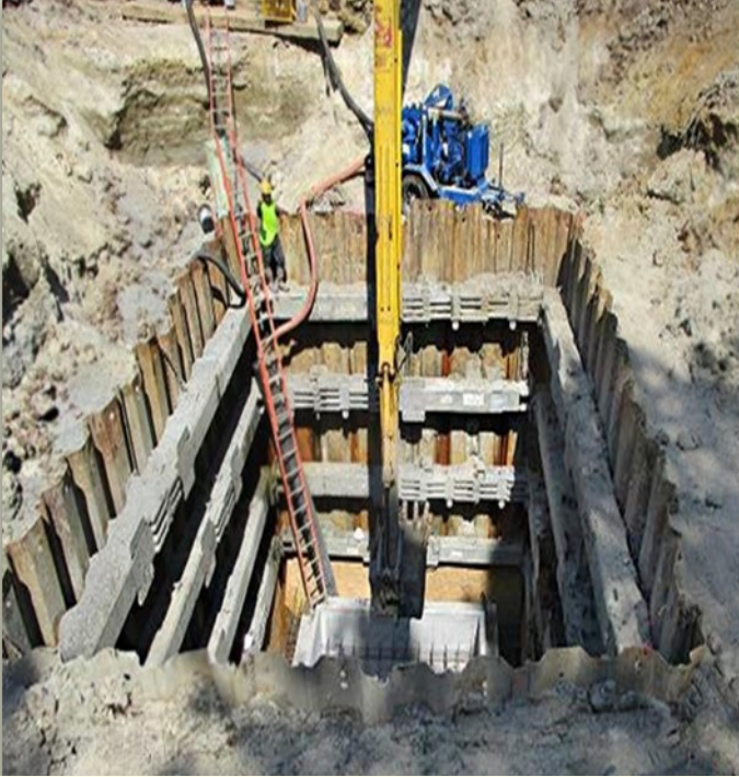
Wet Well Construction
