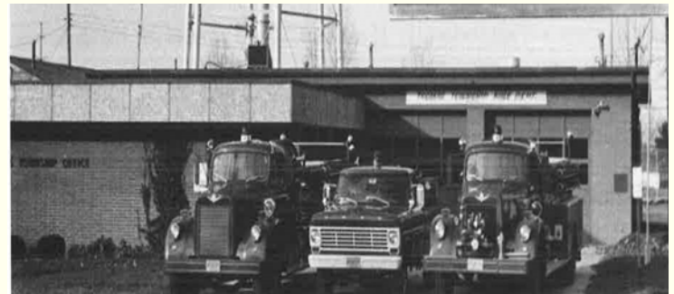
Thomas Township's Fire Station One (North Miller Rd.)
