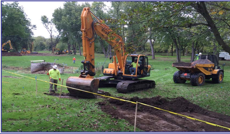
Construction crews excavate 12" of soil from about a dozen backyards along N. River Road south of Dice. The yards are in a floodplain along the Tittabawassee River. Dow Chemical was removing contaminated soil under the direction of the Environmental Protection Agency.
