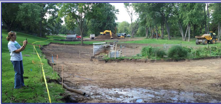
A resident photographs the excavation of 12" of soil from about a dozen backyards along N. River Road south of Dice. The yards are in a floodplain along the Tittabawassee River. Dow Chemical was removing contaminated soil under the direction of the Environmental Protection Agency.
