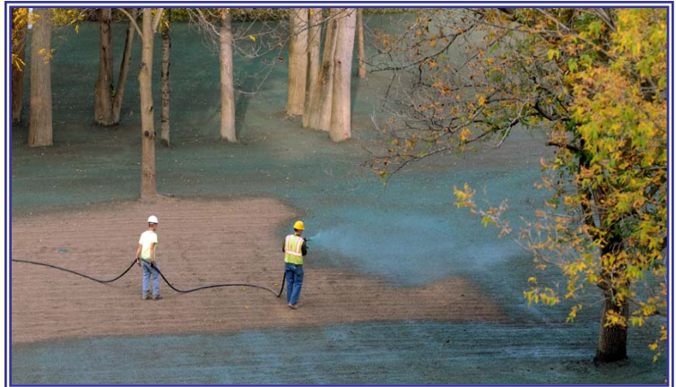
After 12" of soil was removed and replaced with clean soil the yards are seeded. About a dozen backyards along N. River Road south of Dice were involved in the project. The yards are in a floodplain along the Tittabawassee River. Dow Chemical was removing contaminated soil under the direction of the Environmental Protection Agency.
