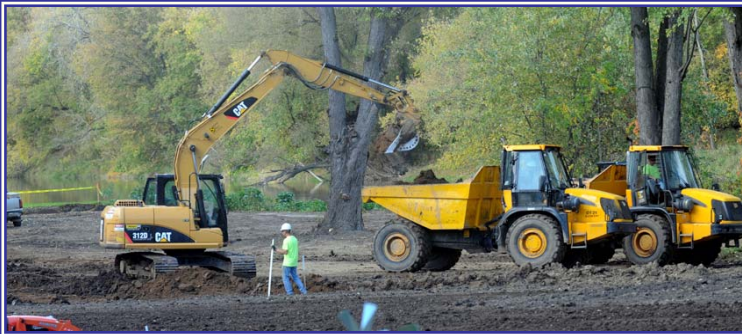
Construction crews excavate 12" of soil from about a dozen backyards along N. River Road south of Dice. The yards are in a floodplain along the Tittabawassee River. Dow Chemical was removing contaminated soil under the direction of the Environmental Protection Agency.
