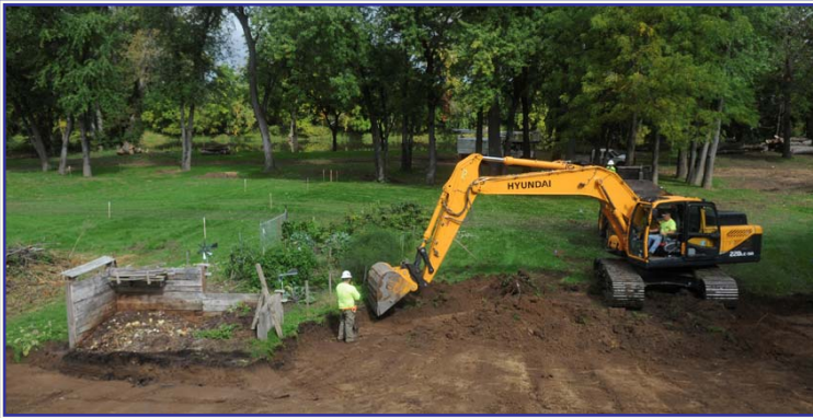
Soil is removed from about a dozen backyards along N. River Road south of Dice. The yards are in a floodplain along the Tittabawassee River. Dow Chemical was removing contaminated soil under the direction of the Environmental Protection Agency.
