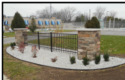
Fencing to be connected to columns directly.
