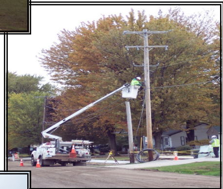
Utility Lines Being Removed
