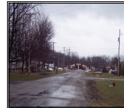
Miller Court Before Work
