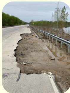
State Road Bridge Damage
